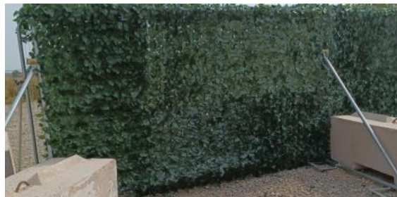
Plate 3.5 Heras fencing with attached textured plastic hedgerow (source: HS2/ EKFB, in Reason, P.F. and Wray, S. (2023). UK Bat Mitigation Guidelines: a guide to impact assessment, mitigation and compensation for developments affecting bats. Version 1.1. Charter
